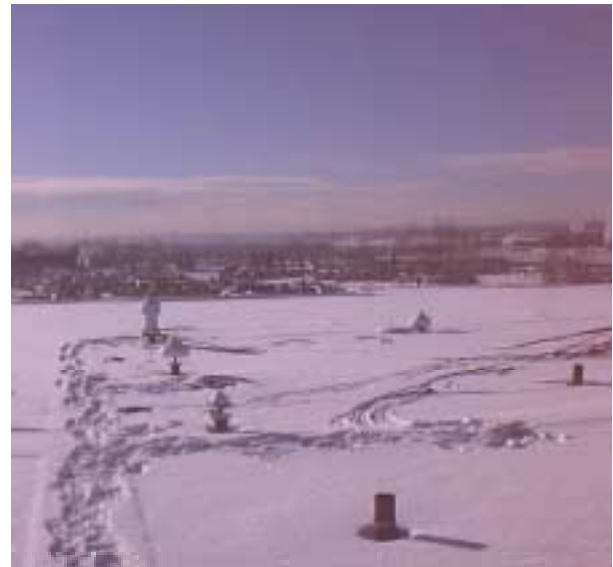
Figure 7: Antenna array on the roof at NovAtel Inc.
