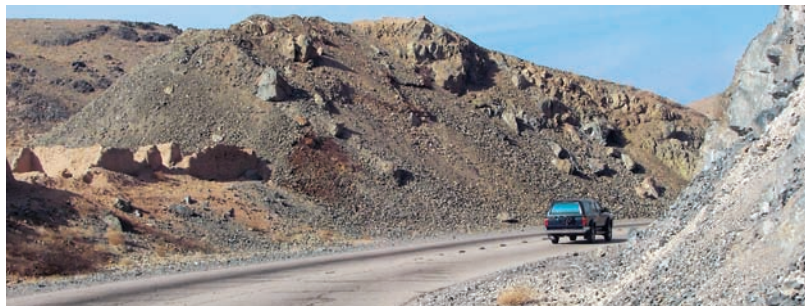
▲ A SECTION of the Kabul-to-Kandahar highway, found to be in better shape than most other segments prior to reconstruction. Travel on other stretches was often limited to 10 kilometers per hour due to poor road conditions.
